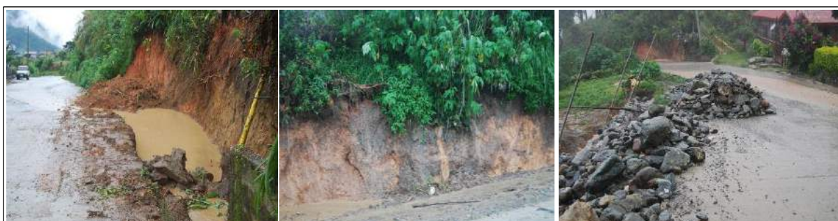
Figure 4.19. Problems prevalent during the rainy season. These photos were taken in June and shows the accumulation of water run-off (left), areas of soil erosion (middle), and the volume of water that runs on the road pavement if the drainages are not put into place (right). The absence of parapet walls/retaining walls allow for landslides to happen.
