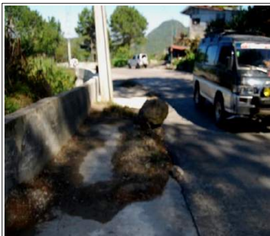
Figure 2.28. A boulder obstructing part of the emergency bay (x=267,973 m, y=1,860,036 m, elevation = 1,652 m)
