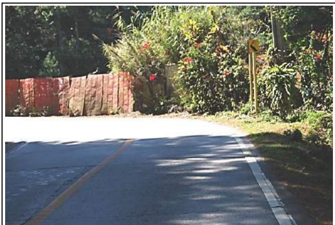
Figure 2.27. Barriers with no reflective materials (x=264,304 m, y=1,865,868 m, elevation = 1204 m)
