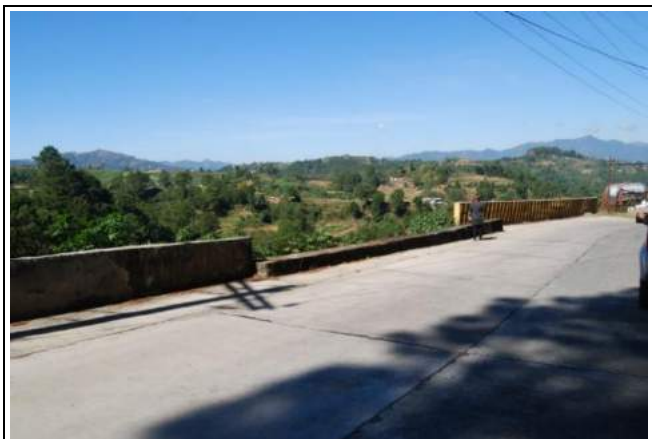
Figure 2.26. Inconsistency of guardrail designs (x=267,980 m, y=1,860,229 m, elevation = 1625 m)
